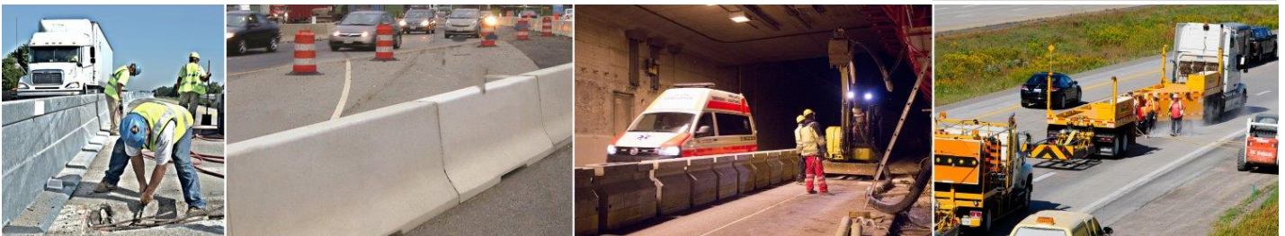
Positive Protection Barriers provide separation and help prevent longitudinal and lateral crashes into work zones.
